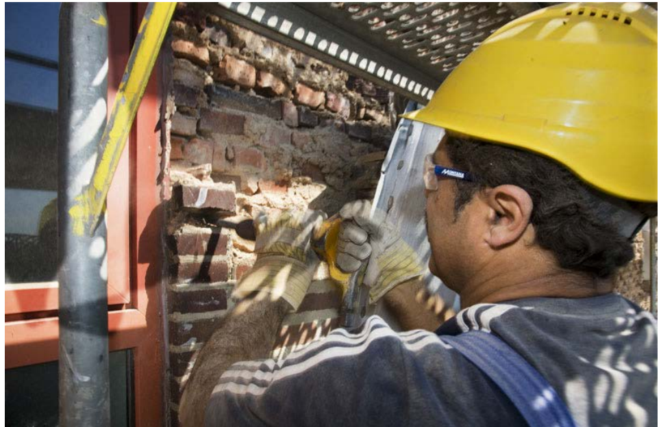
Figure 61 Hand removal of the brickwork and demolition of the western annexe building
