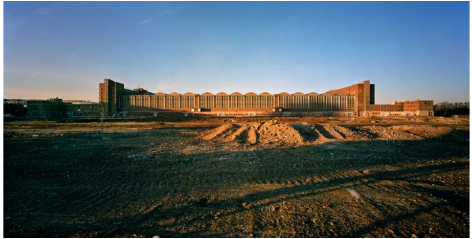
Figure 2 120,000 m 2 entire site area
