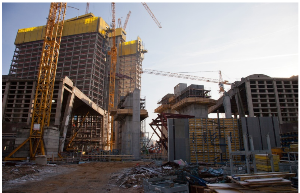
Figure 69 Foundation work for the Entrance building
