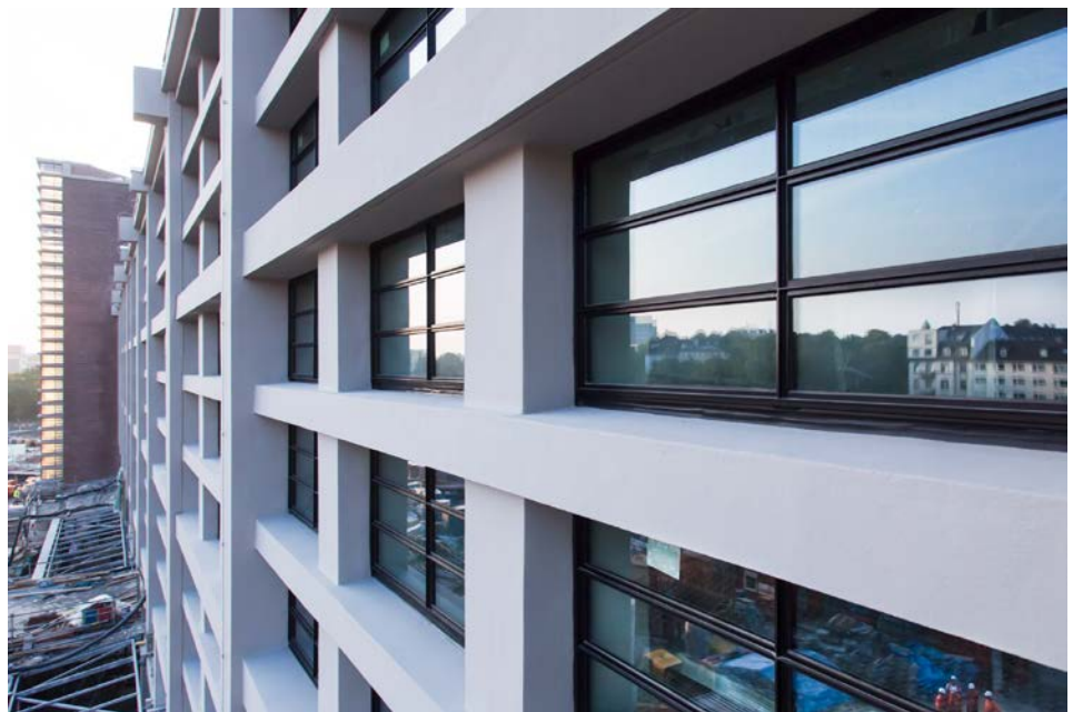
Figure 3 250 m long Grossmarkthalle
