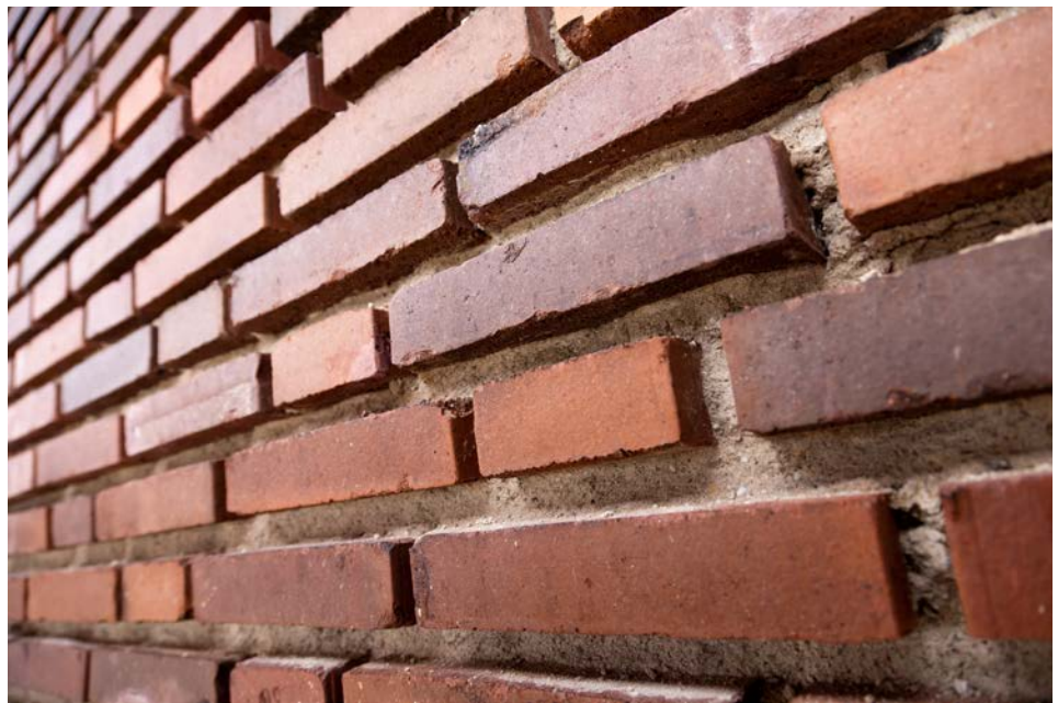
Figure 4 73 km of restored joints
