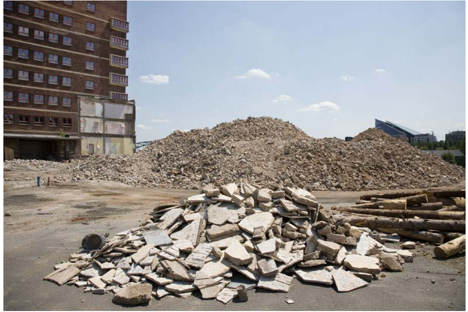
Figure 61 Hand removal of the brickwork and demolition of the western annexe building
