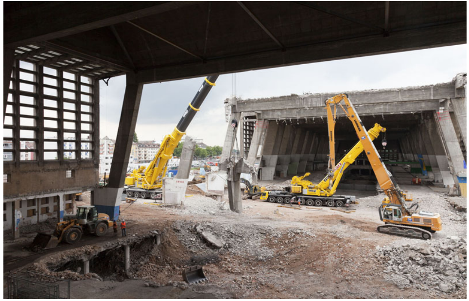
Figure 68 Removal works Entrance
