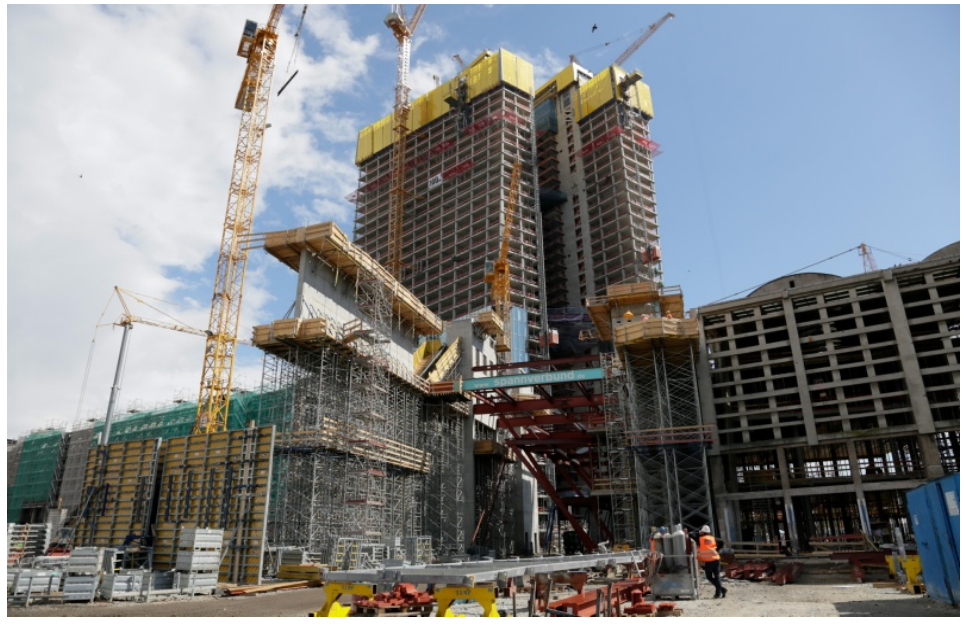
Structural framework for the “house in house” building elements
